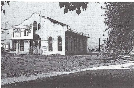
Ivy Substation - Monument #182
